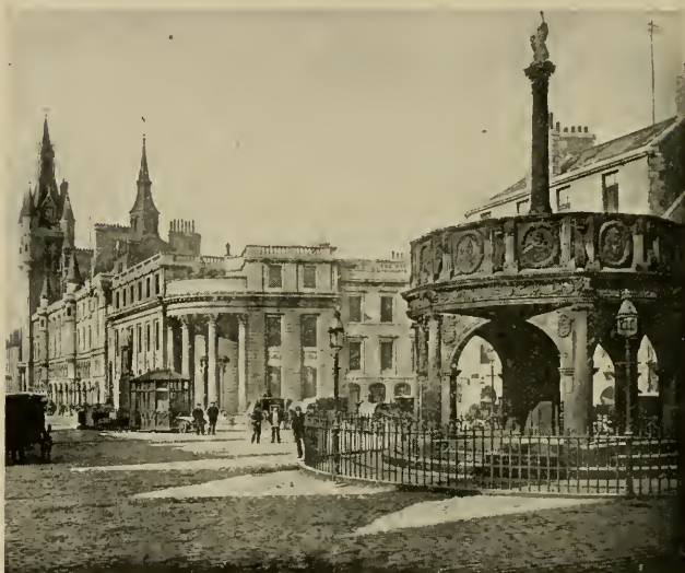
Municipal Buildings, Aberdeen, and Town Cross
